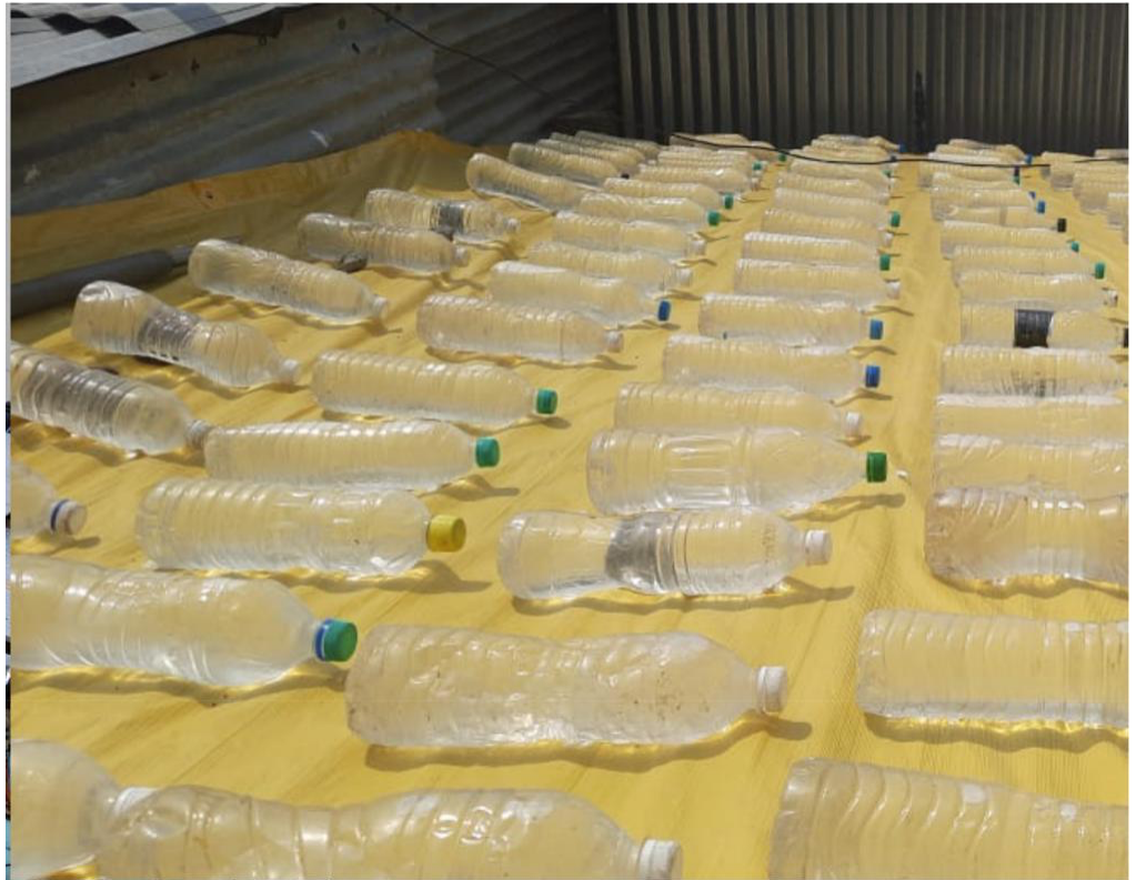
Plastic bottles filled with water which absorbs the sun's heat, keeping the building cool for longer (Image: cBalance)
